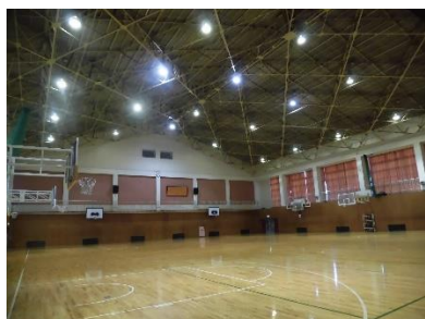
[LED照明工事前]
