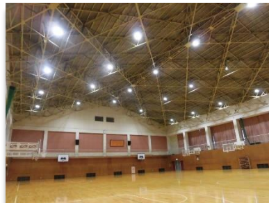
[LED照明工事後]
